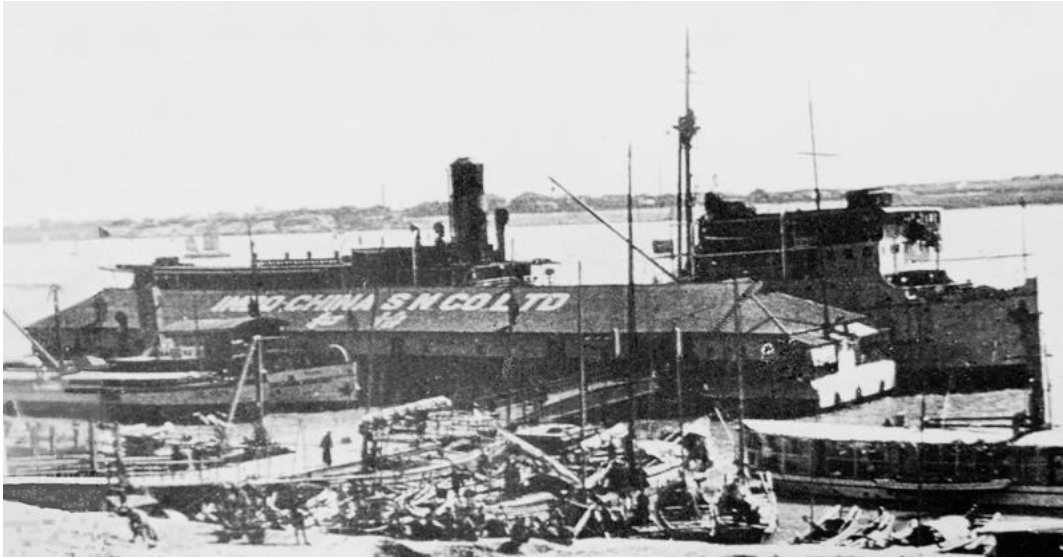
PING WO at Hankow in 1930s. Superstructure now closed in forward and extended aft, but still with a trunked cargo hatch ( China Proper Vol III , UK Naval Intelligence, 1945).
