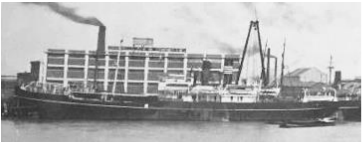
Likely MING SANG at the New Engineering & S.B. Co. yard in Shanghai (New E.& S.B. Co.).
