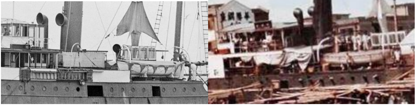
Comparison of superstructure sections of prewar and postwar photos, showing convergence.
