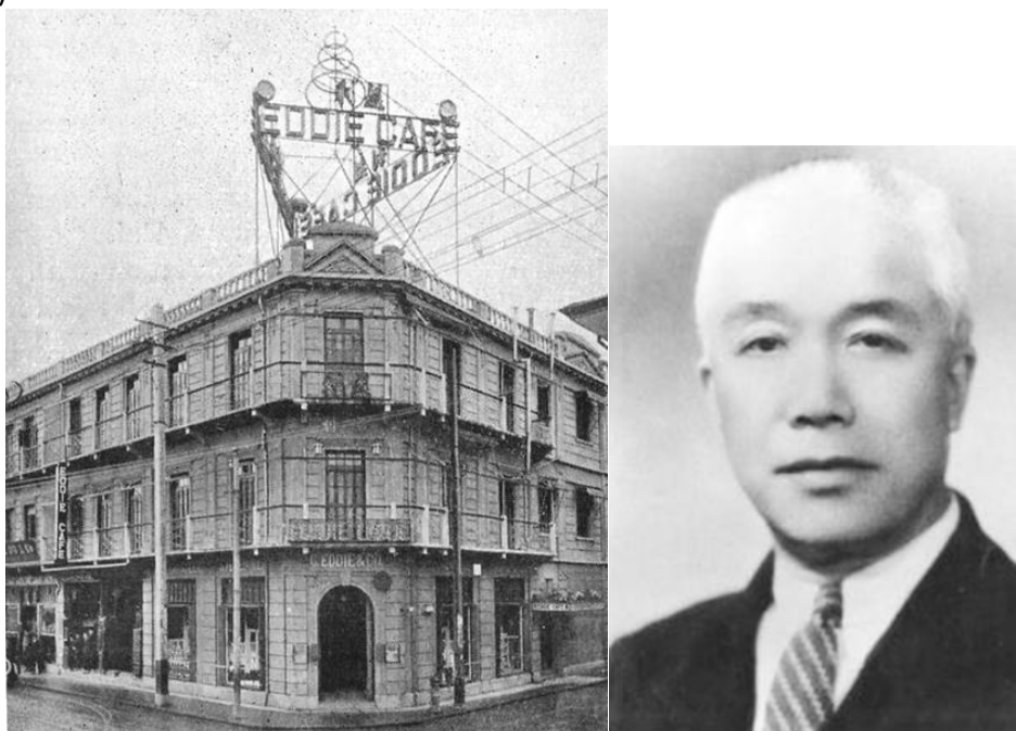
C. Eddie Hsu and C. Eddie & Co. building in early 1920s with Eddie café on the ground floor and prominent neon signage (York Lo, 2019)
