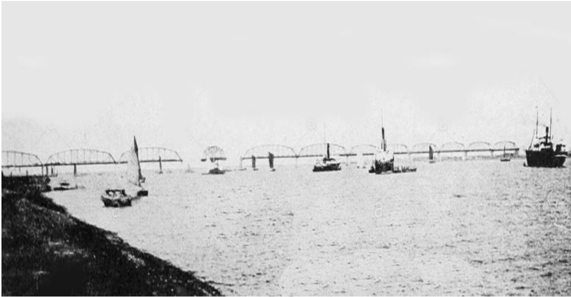
The Yalu bridge with the swing span (Internet).
