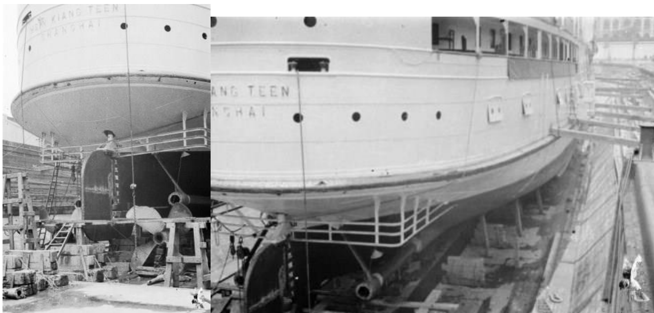
Built up stern, propeller blades under repair, Shanghai 1937 (Harrison Forman, UWM Libraries).
