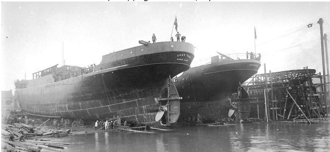
PROSPER (#554) middle hull) under construction at Kowloon. Nearside vessel is somewhat larger CHAK SANG (#553) of Indo-China S.N. Co. The third vessel would be HERMELIN (#548) (HK&WD/HKMM ID 2008.0197.019b).
