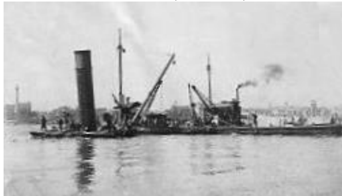
HANYANG under salvage (Internet).
