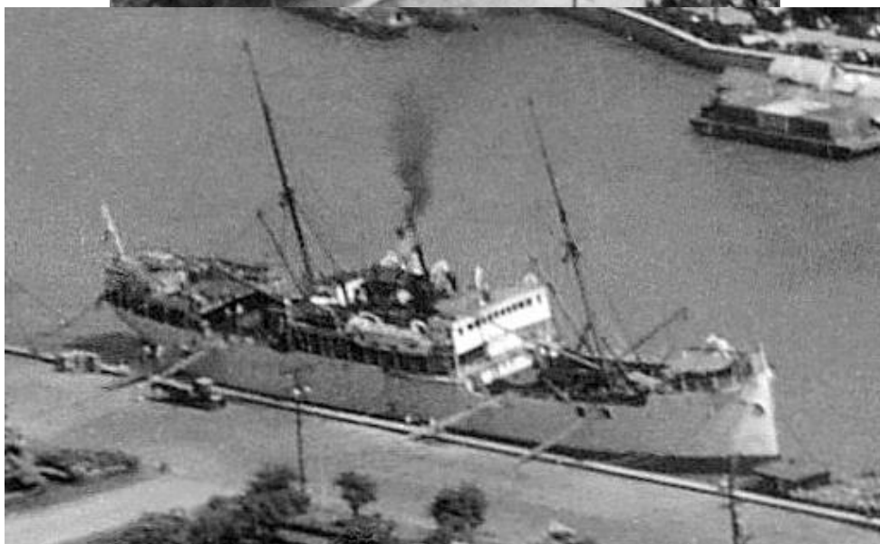
Above 2: MAUBAN 13 July 1936. Awning removed at poop (USNA/John Tewell).
