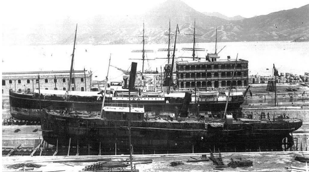
PEDRO DE SOTOLONGO at Taikoo Dockyard 2010 after lengthening and plating in of the well deck but prior to renaming as UNION, CNC's Nanchang on other side (HKMM).
