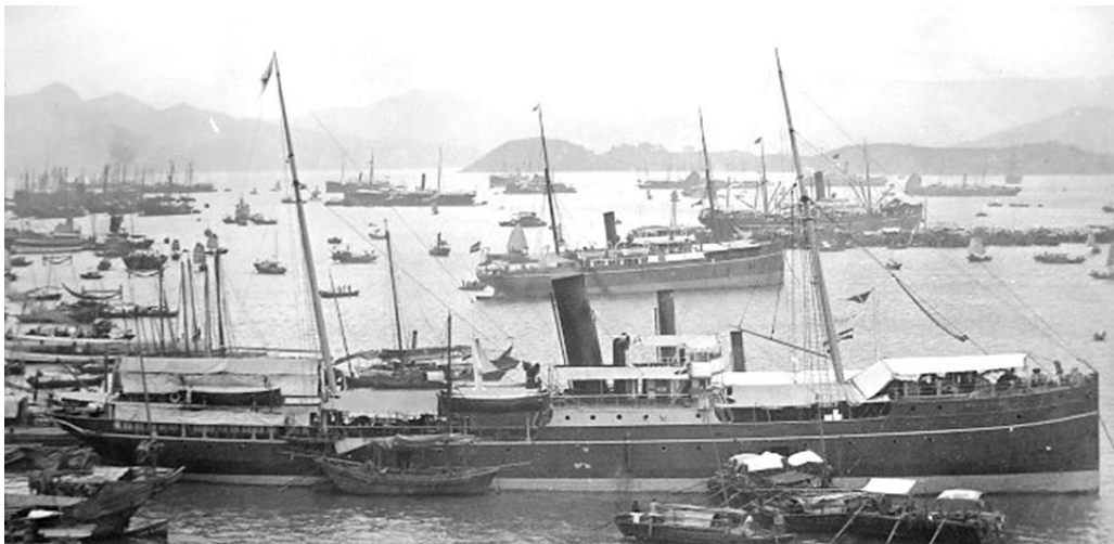
HAILOONG at DSSC wharf, late 1890s (HKMoH*).
