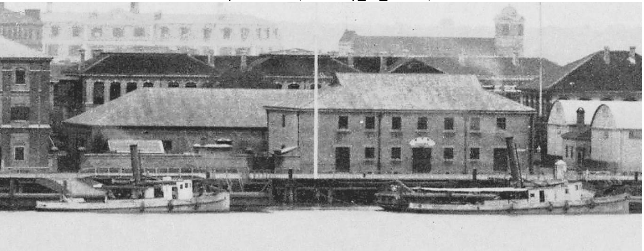
Two small unidentified tug-tenders with barges at the Nippon Yusen Kaisha (NYK) wharf at Nantao in an 1898 Kung Tai panorama (Royal Commonwealth Society/UofCambridge).
